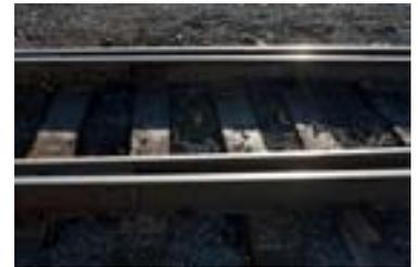
The foundation beneath, including ballast, ties and plates, helps keep the rail in place with as little movement as possible.
