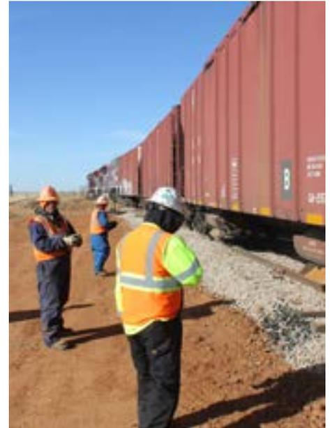
IPH General Roadmaster Randall Roberson, foreground, assists Balfour Beatty Rail crews in unloading ballast rock from the unit train onto newly built tracks at the Levelland facility.
