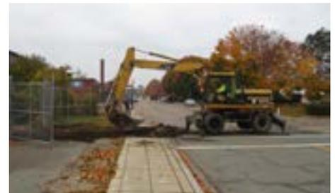
A crossing is torn out on Water Street, near the Fall River, Mass., wharf at the beginning of a rebuilding project. Water Street needed rail enhancements as the road has become the main detour route during the Highway 79 bridge reconstruction, which is over top of Mass Coastal's track.
