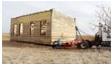
**ABOVE:** Neudorf Construction uses a winch truck to jack up the Whiteface depot in preparation for its move to Wolfforth, Texas. **LEFT:** The Whiteface, Texas, depot, pump house and water tank serve trains on the Panhandle and Santa Fe Railway. Photo circa 1931.
