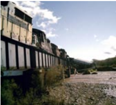
AZER employees and contractors worked diligently to clean up the damage.
